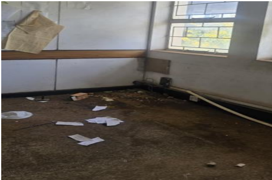
Figure 3: Old nutec board partitions and polyester carpet to be removed
